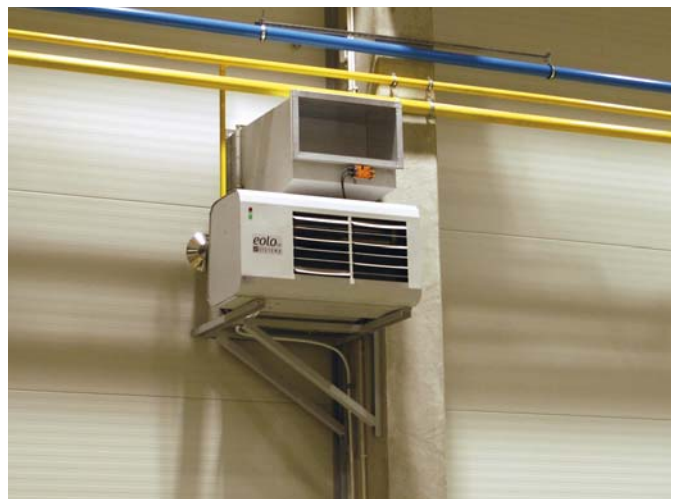
EXTERNAL-INTERNAL AIR RECIRCULATION WITH AIR DAMPER
