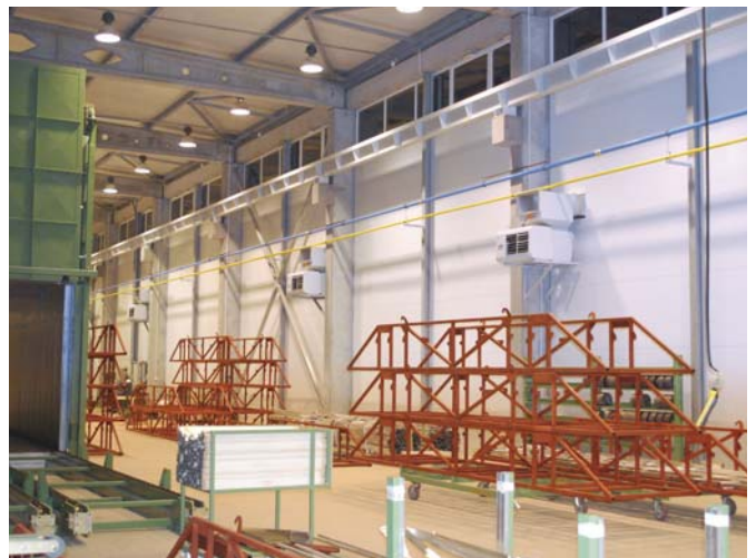
EXTERNAL-INTERNAL AIR RECIRCULATION WITH AIR DAMPER
