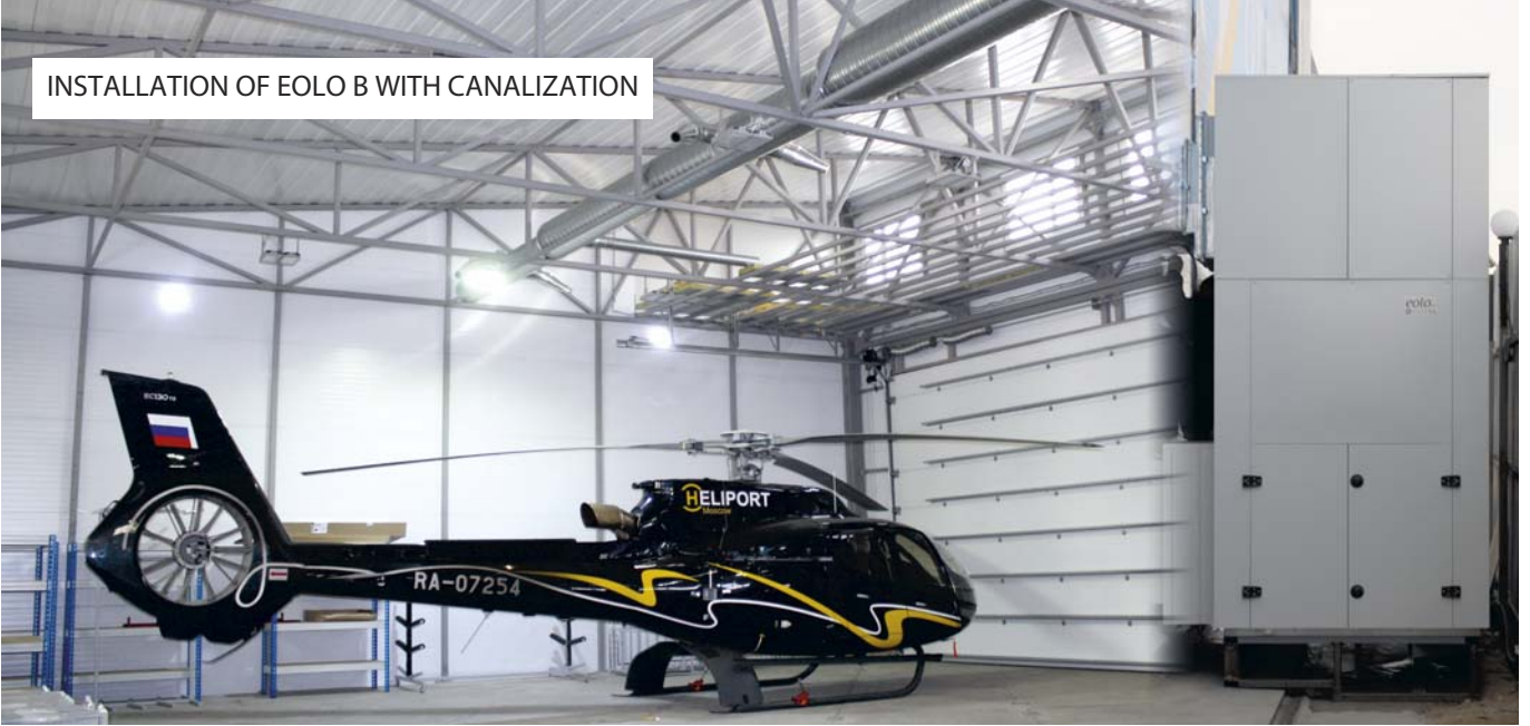
INSTALLATION OF EOLO B WITH 2 WAYS DUCT
