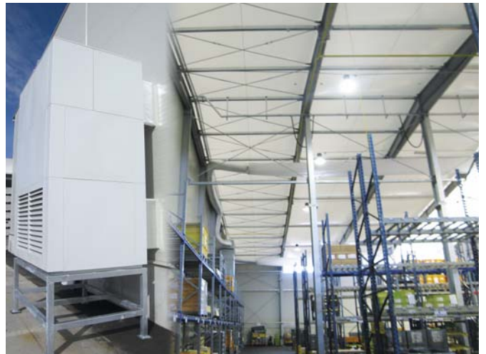
INSTALLATION OF EOLO B WITH CANALIZATION
